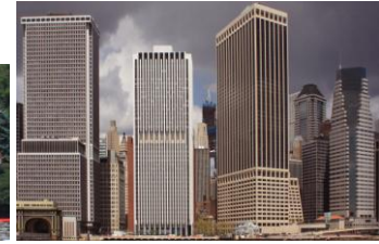
Battery - 2 Parts - 10.5h x 16w
